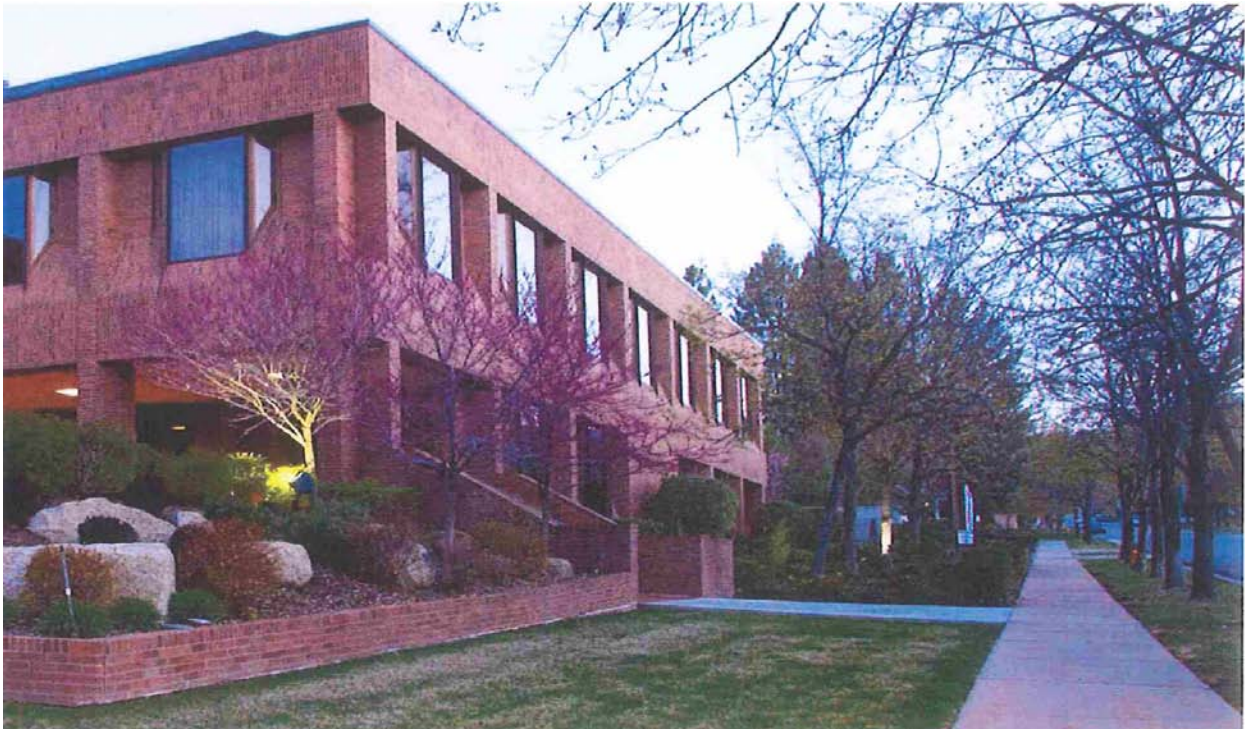
Exterior of building looking north on J Street.
