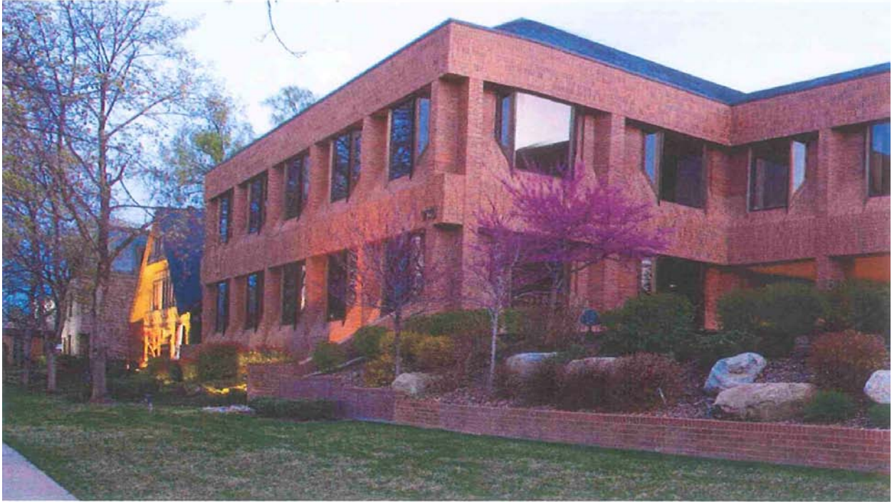
Exterior of building facing South Temple Street
